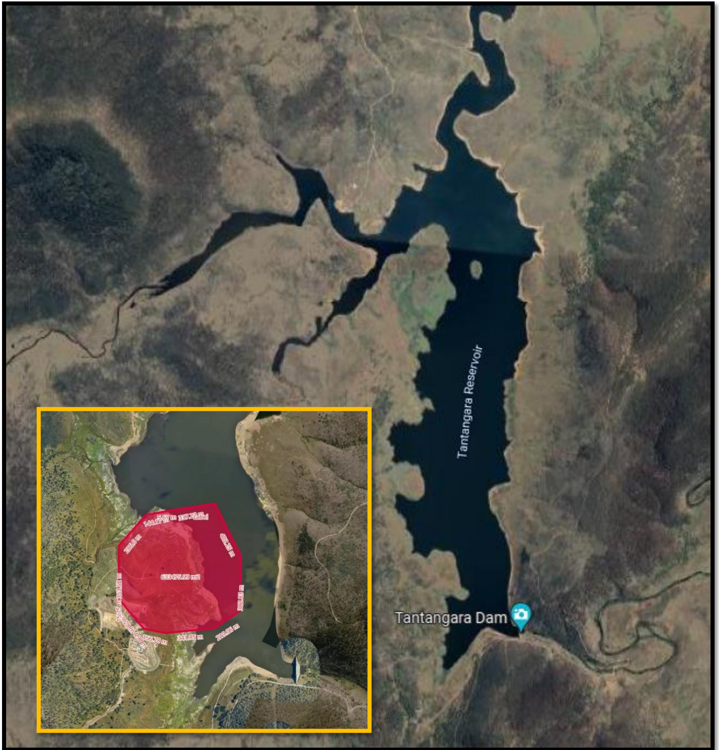
Blast area from Snowy 2.0 worksite at southern end of Tantangara Reservoir
